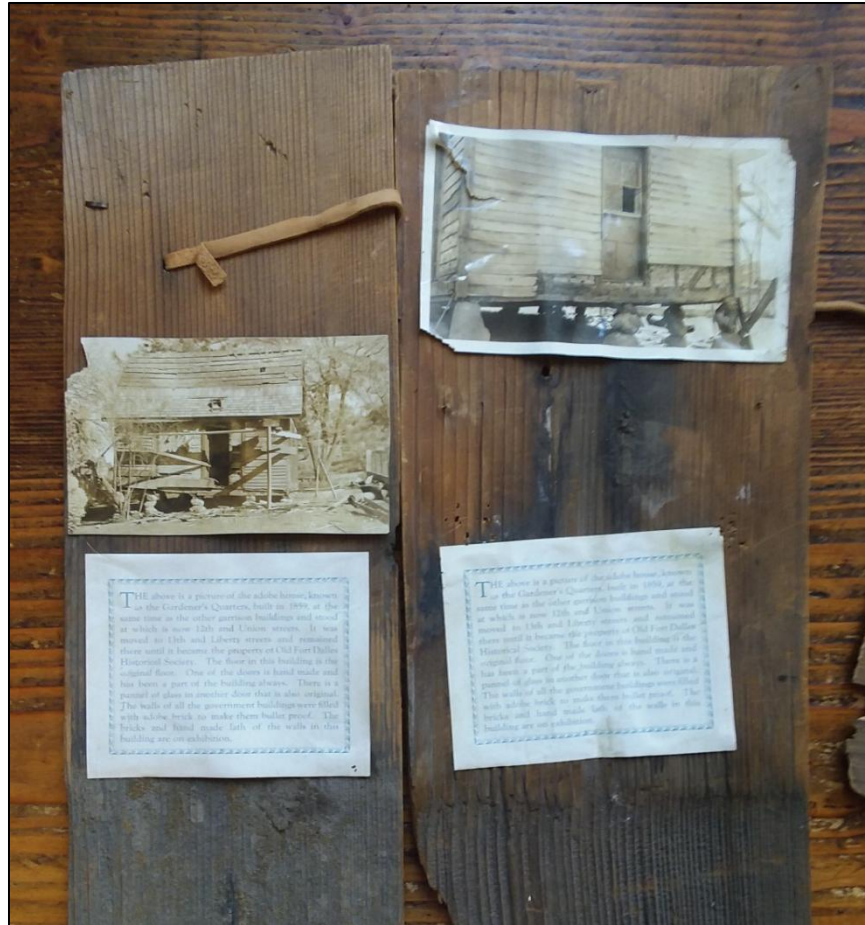
FIGURE 9: ORIGINAL SHINGLES FROM THE GARDENER'S COTTAGE, IN THE FORT DALLES MUSEUM COLLECTION. PHOTOS SHOW THE RELOCATED BUILDING.
