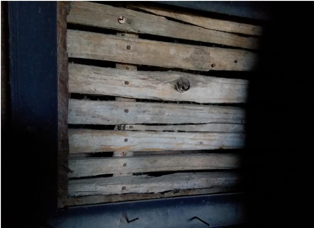
FIGURE 16: DISPLAY FRAME SHOWING HAND SPLIT LATH ON INTERIOR WALLS.
