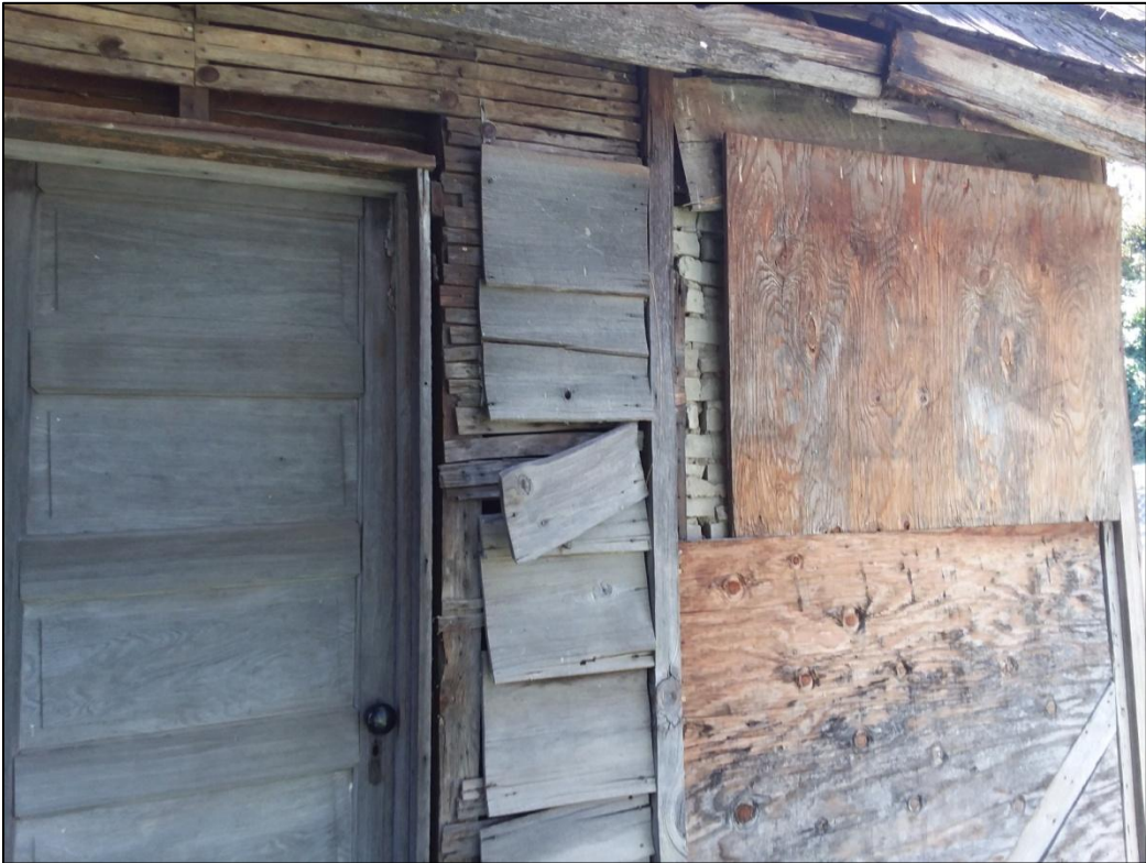
FIGURE 18: WESTERN EXTERIOR WALL SHOWING LATH, AND BRICK INFILLING.
