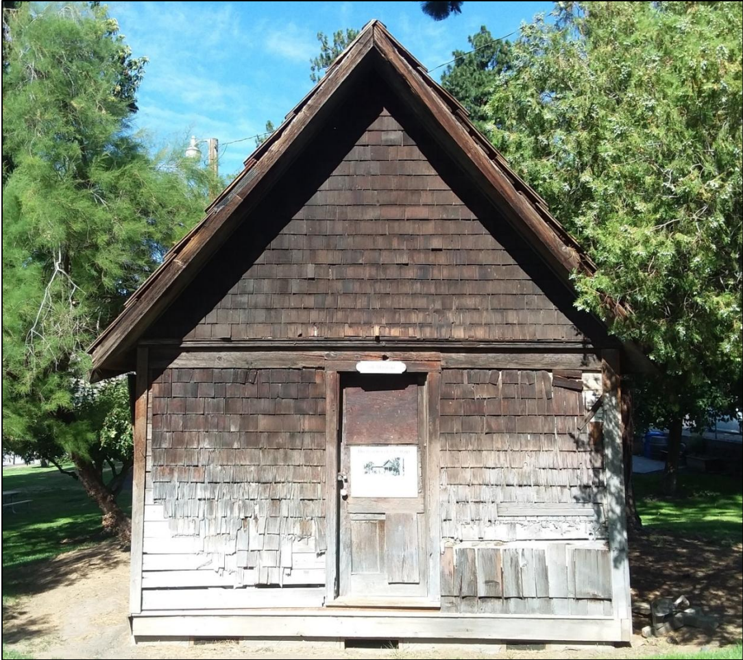
FIGURE 4: SOUTHERN WALL OF THE GARDENER'S COTTAGE AT FORT DALLES MUSEUM.
