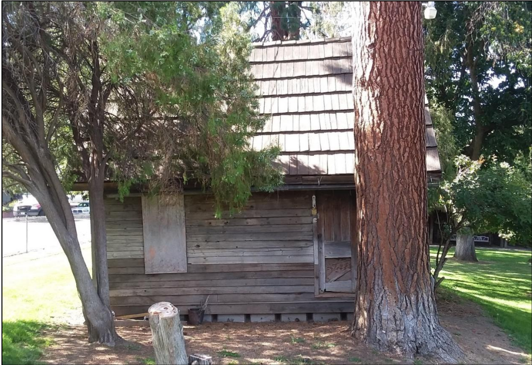
FIGURE 7: EASTERN WALL OF THE GARDENER'S COTTAGE, FORT DALLES MUSEUM.
