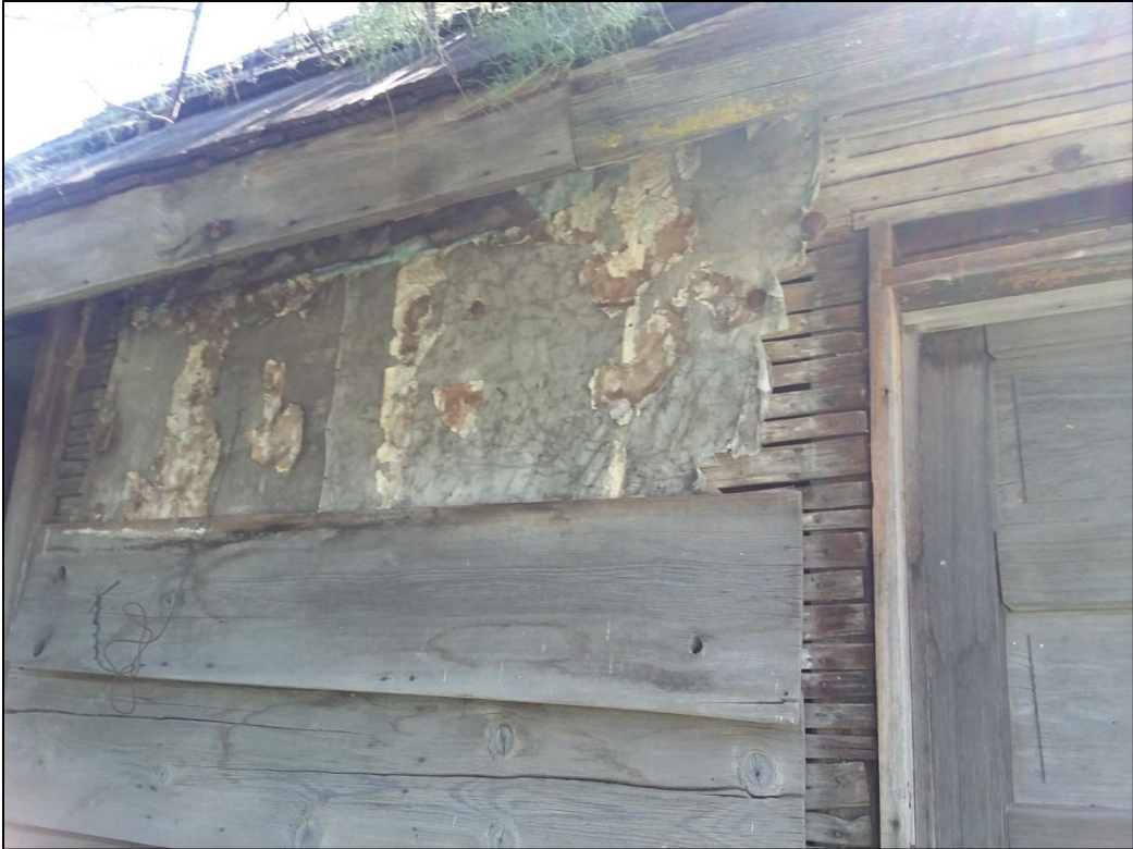
FIGURE 17: WESTERN OUTSIDE WALL SHOWING LATH AND MUSLIN BACKED WALLPAPER ON WHAT WAS AN INTERIOR WALL.
