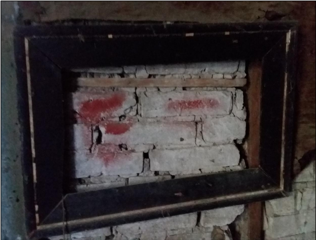
FIGURE 15: DISPLAY FRAME SHOWING BRICK INFILLING OF EXTERIOR WALLS.
