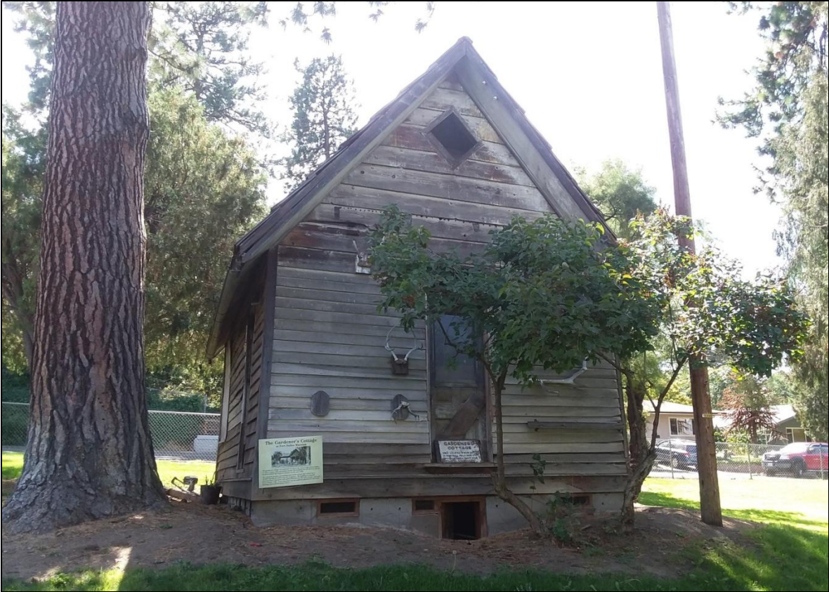
FIGURE 6: NORTHERN WALL OF THE GARDENER'S COTTAGE, FORT DALLES MUSEUM.
