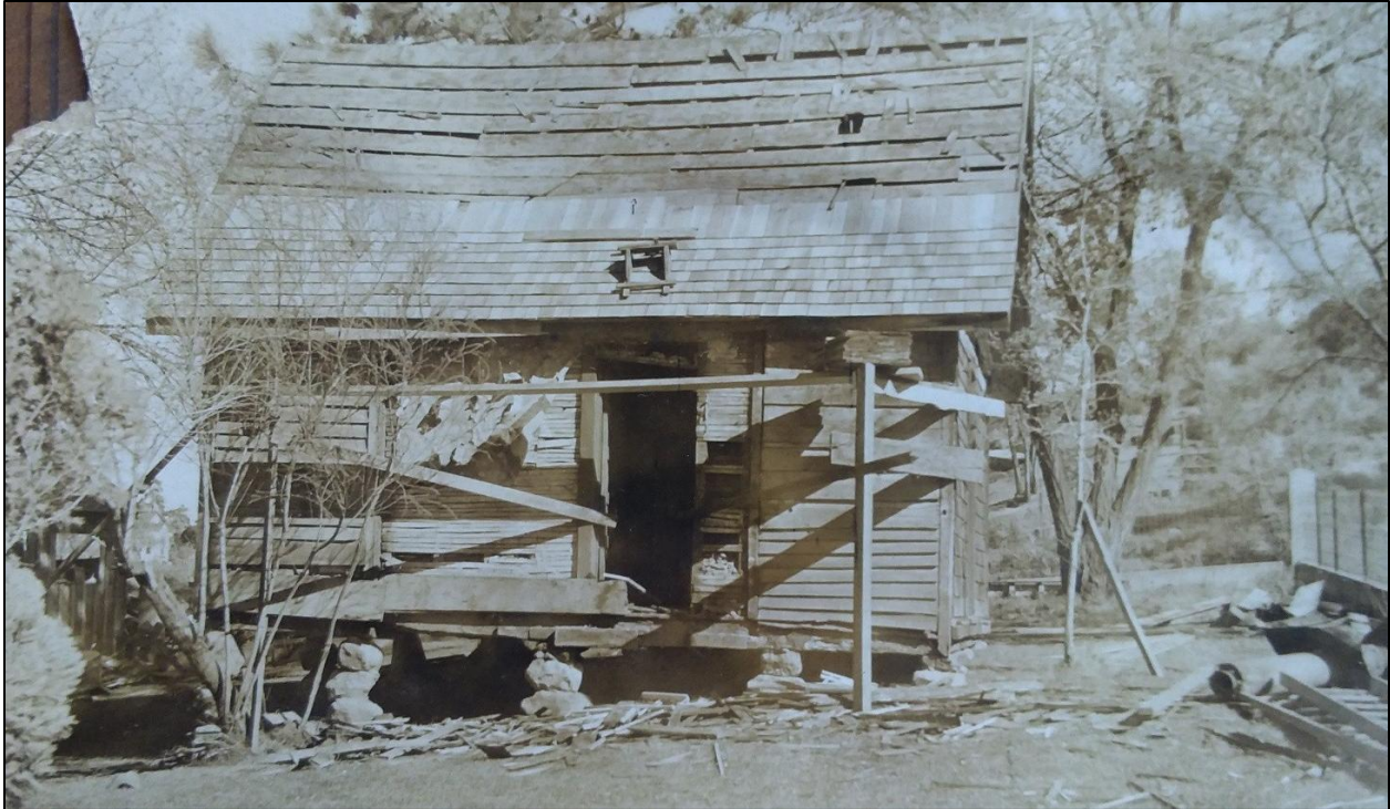
FIGURE 11: EASTERN SIDE OF GARDENER'S COTTAGE AFTER THE 1930S MOVE.
