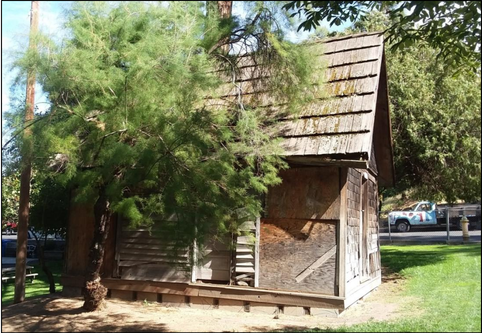
FIGURE 5: WESTERN WALL OF THE GARDENER'S COTTAGE, FORT DALLES MUSEUM.
