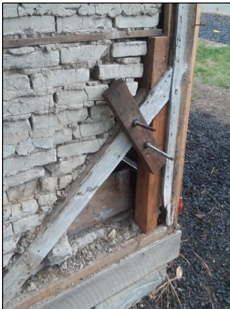
FIGURE 3. SW CORNER SHOWING CLAMP USED TO MOVE THE CORNER BRACE BACK INTO PLACE AND THE REPLACED BRICK INFILL PRIOR TO PUTTING ON THE PLYWOOD SHEATHING.
