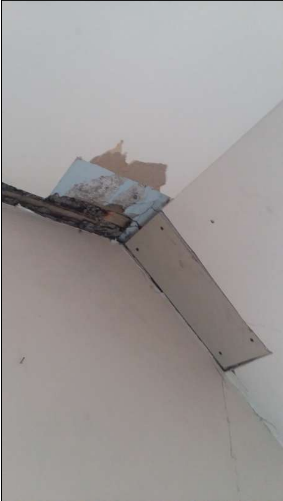
Figure 11: Starting the drywall repairs in the south bedroom.
