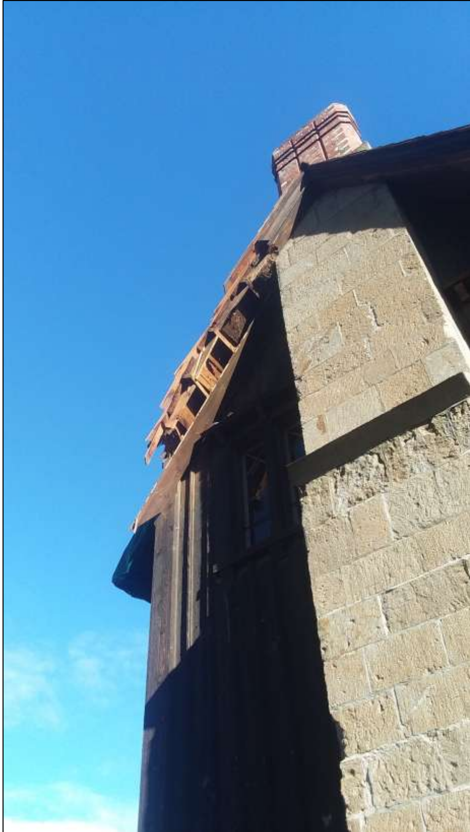
Figure 2: Damaged eave.
