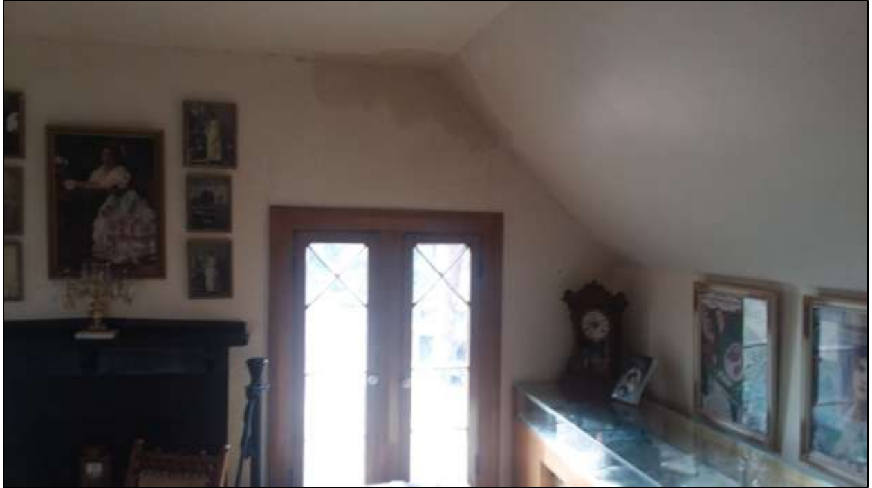
Figure 12: Drywall repairs nearly complete.
