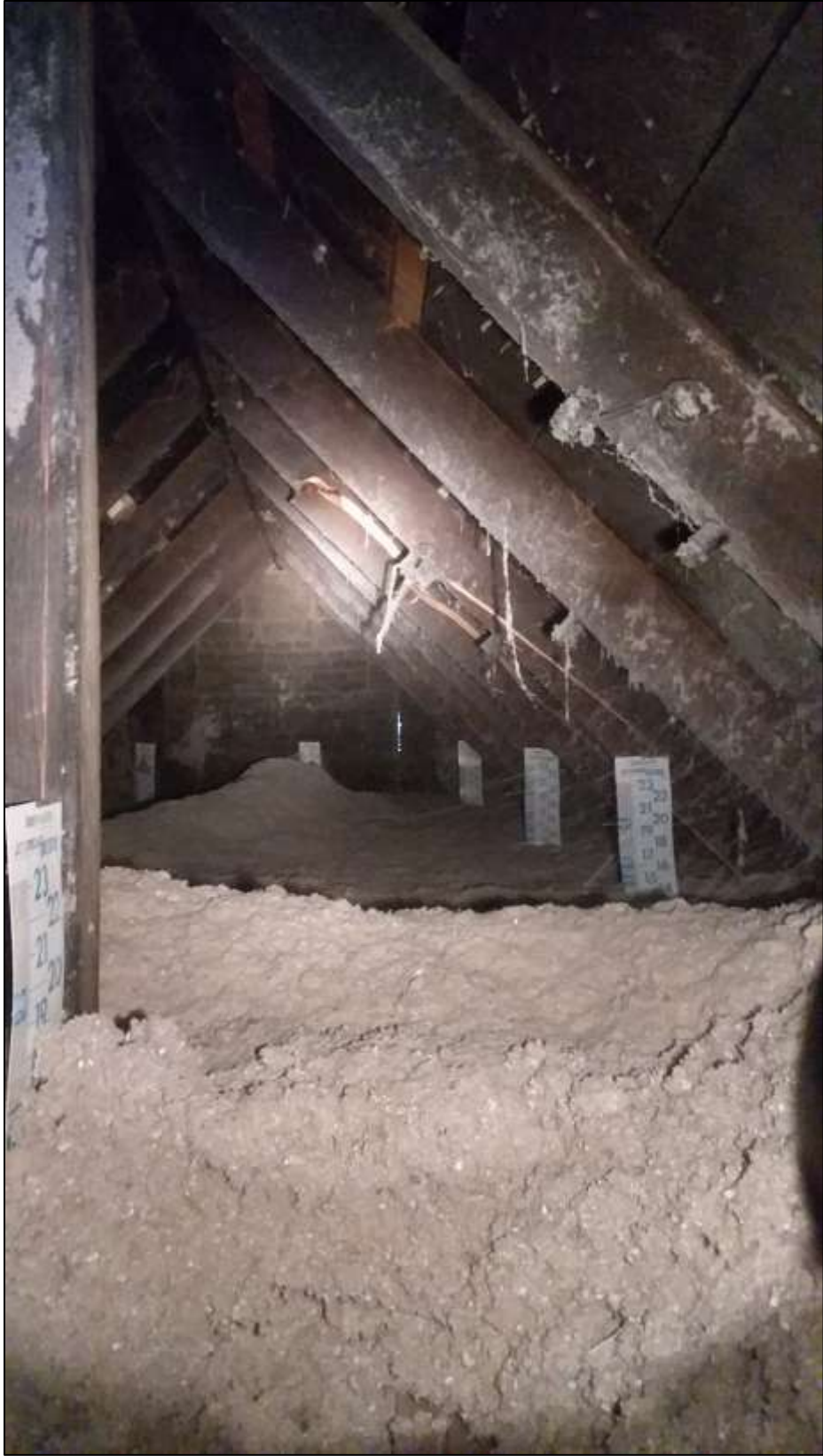
Figure 3: Damaged rafters.
