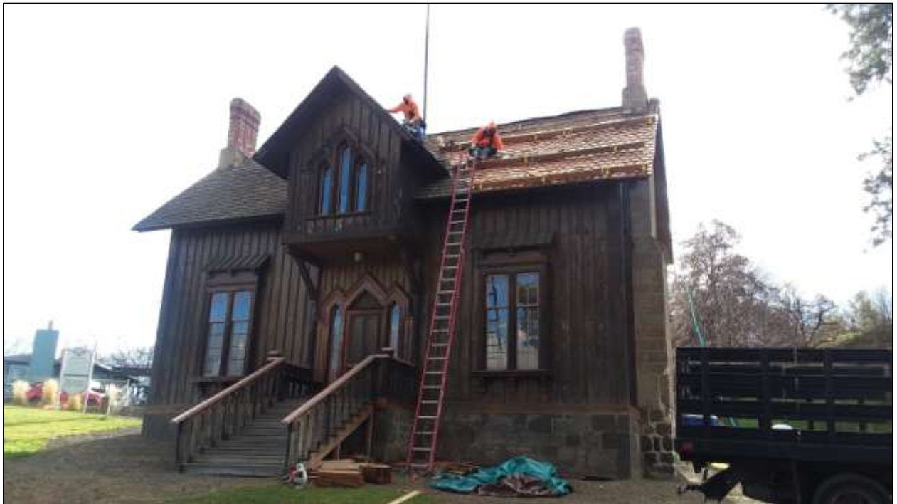
Figure 13: The crew from Brown Roofing repairing the roof.
