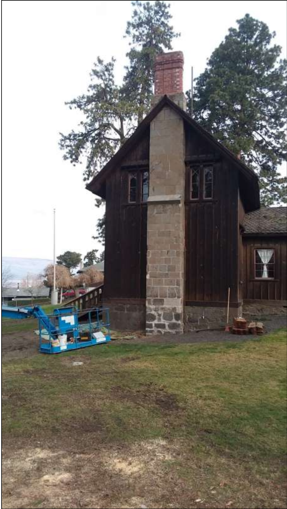
Figure 6: Completed eave repairs.
