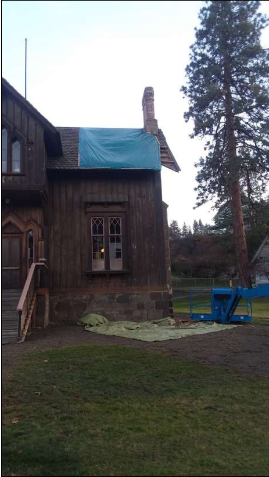
Figure 5: Partially repaired eave.
