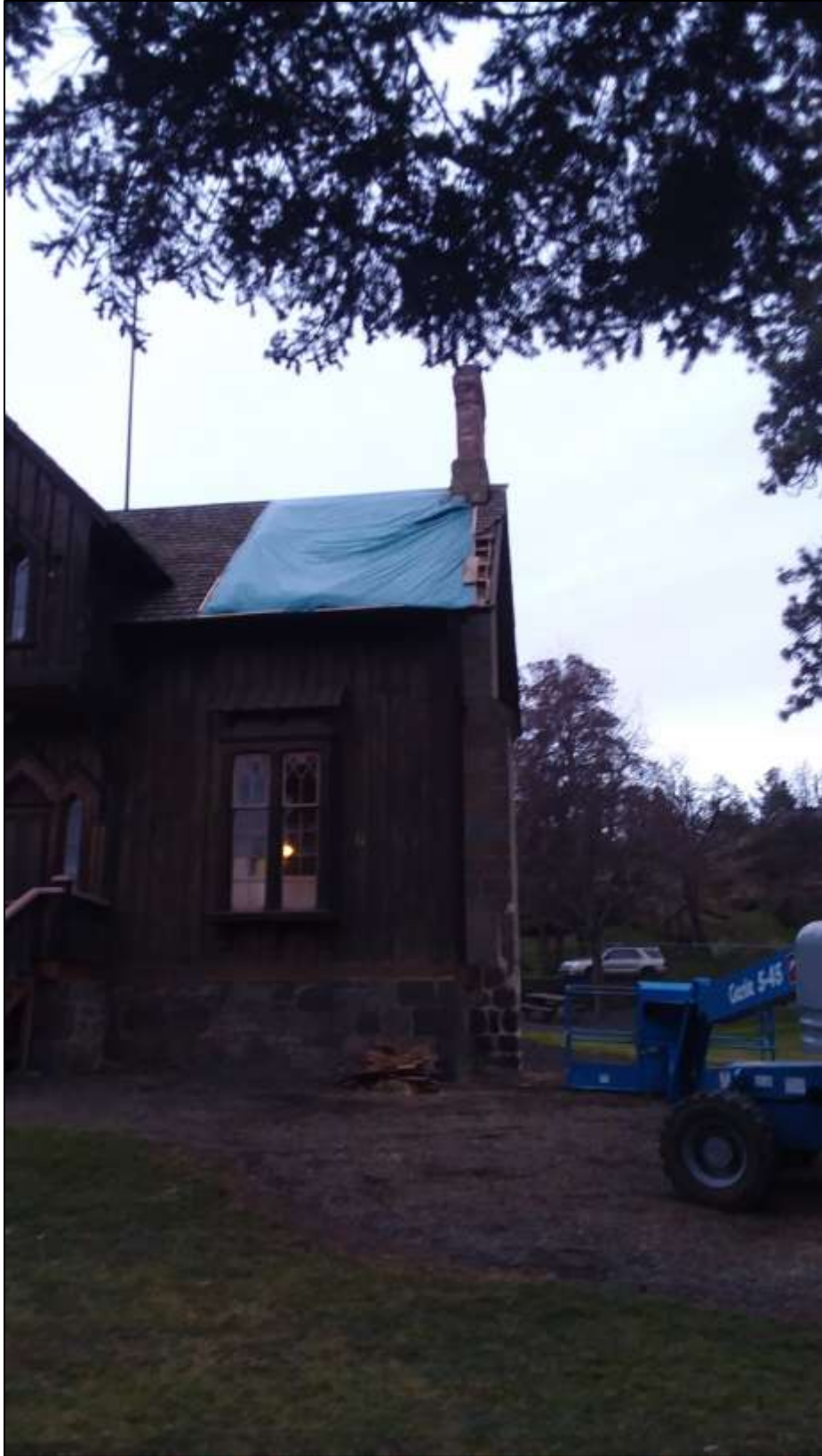
Figure 7: Completed eave repairs.
